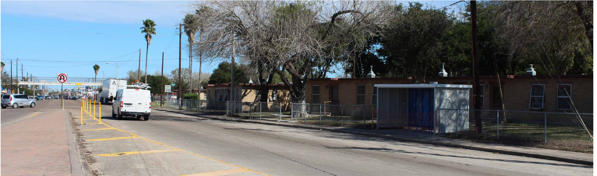
NEW BUS SHELTER ON INTERNATIONAL BOULEVARD LOOKING NORTH
