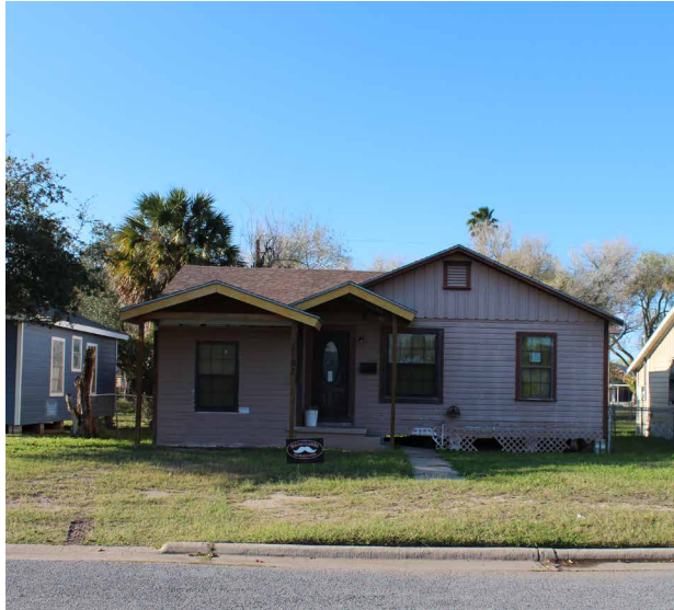
SINGLE FAMILY HOUSING ON 19TH STREET
