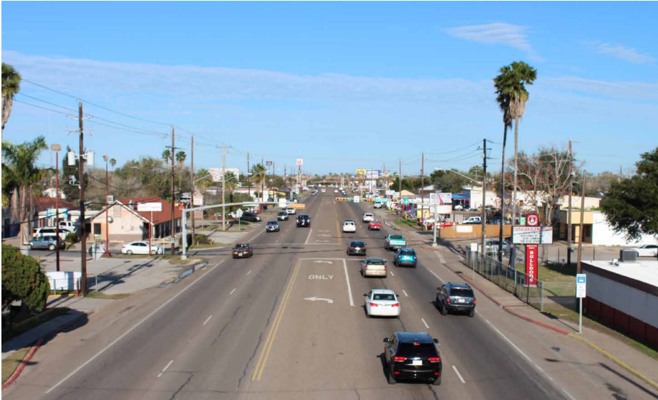
INTERNATIONAL BOULEVARD & GARFIELD STREET LOOKING NORTH
